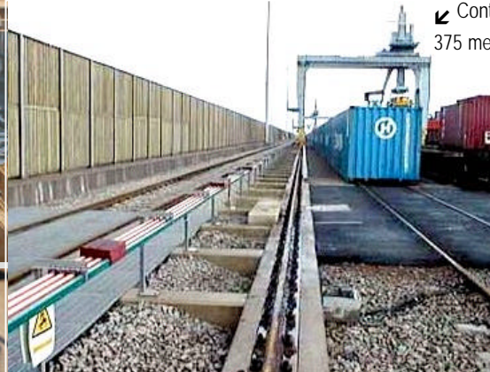
← 3 cranes operating outdoor on a 456 metres system, comprising 3 x 1250A Phase and 1 x 800A Earth conductor.
