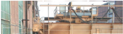
← 3 cranes operating outdoor on a 456 metres system, comprising 3 x 1250A Phase and 1 x 800A Earth conductor.
